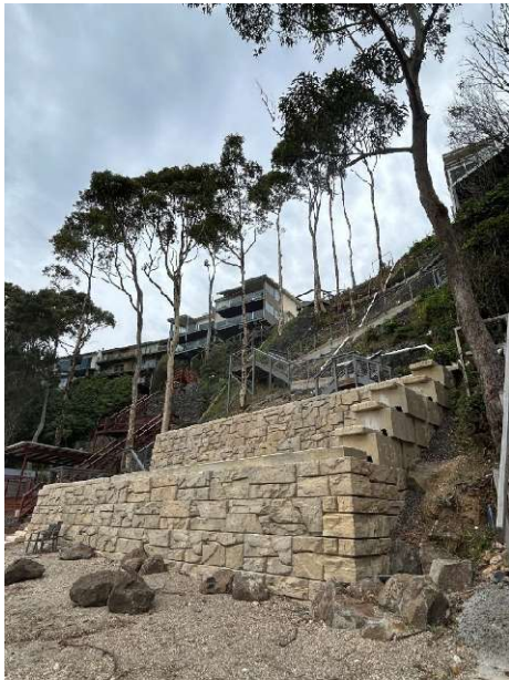
Figure 9: A site photo from 3/12/24 showing as-built works
