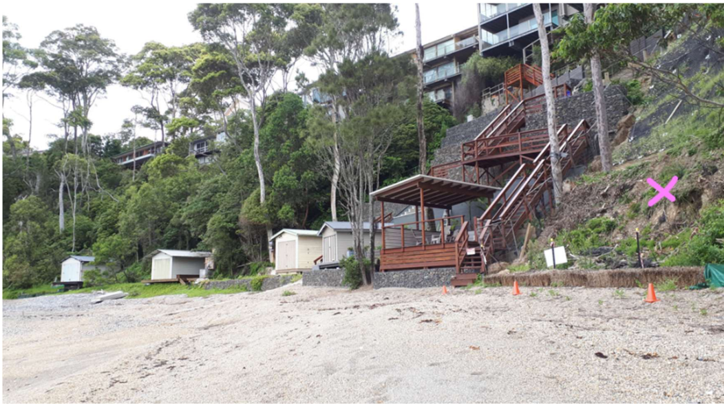
Figure 4: A photo from 20/2/24 showing base of cliff i.e. tidal ocean wave area (looking south)
